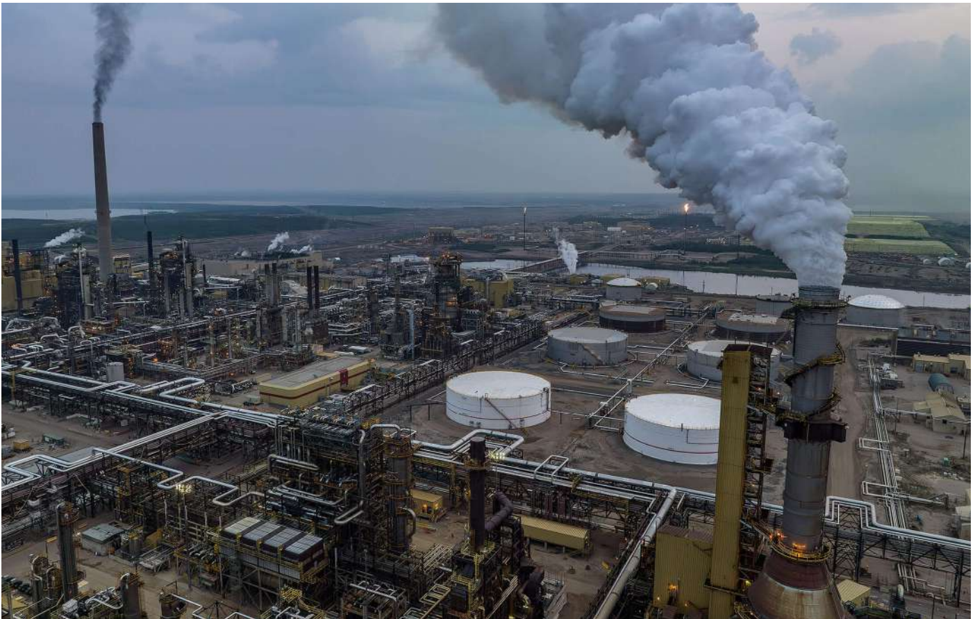
Tar sands processing facility in Alberta, Canada © Markus Mauthe / Greenpeace
